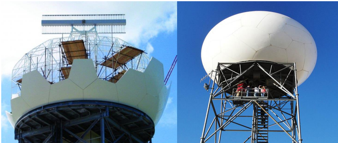
Figure 19 - (Left) Uncovered radar, (Right) Radome covered radar (Military systems and technology, 2010)
